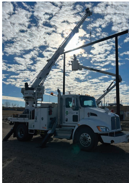
Hanging the entrance gate.
