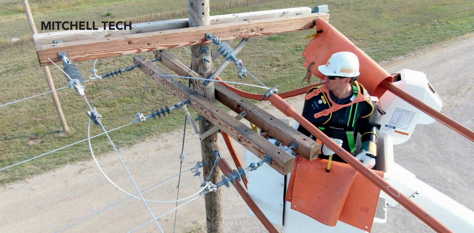
Mitchell Tech facilities were used for the annual electric cooperative rubber gloving school last summer. Photo by Billy Gibson
