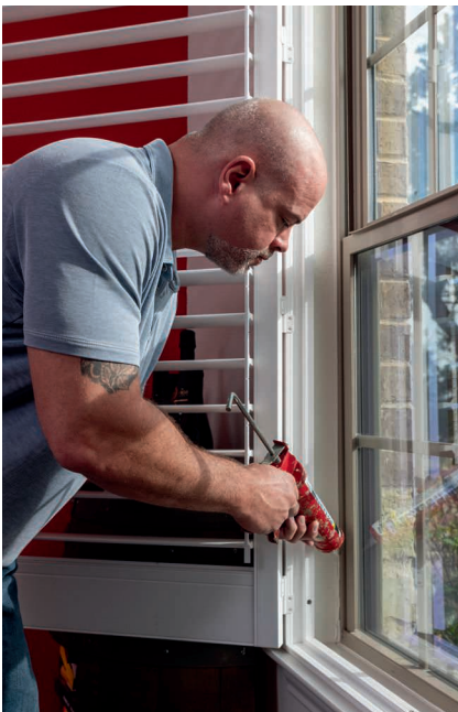
Sealing air leaks around your home is a simple, effective way to save energy and lower your bills.
